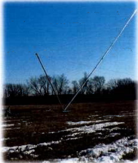
A 199-foot temporary wind test tower was installed to gather wind speed data to assess the feasibility of erecting a permanent wind turbine to power local businesses and homes.
